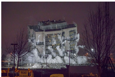
Demolition at Nall Ave & I-435
